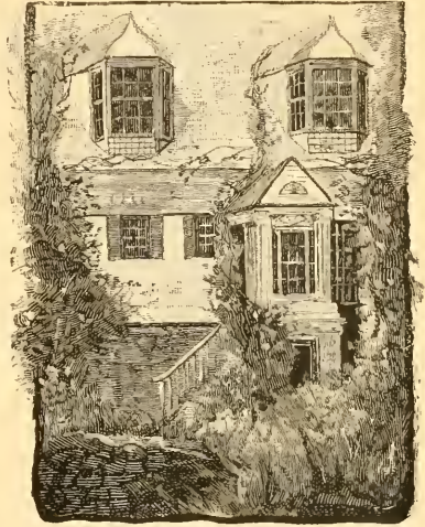
An Old Cottage at Arichat.
